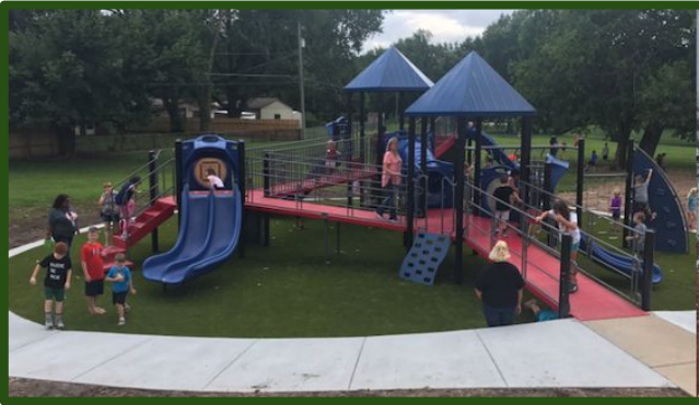
Swaney Elementary received new surfacing and a sidewalk for their ADA accessible playground!
